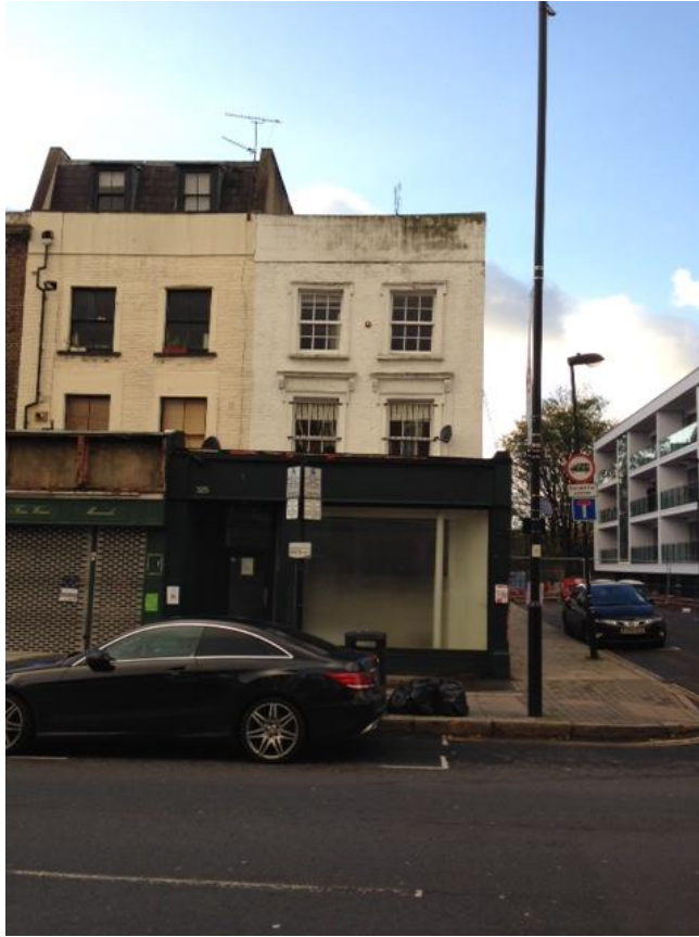
Image 2: View looking west at 325 Caledonian Road.
